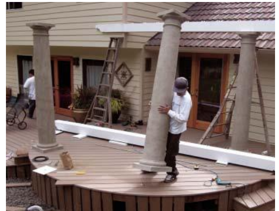
Figure 8. Fiberglass arbor and pergola kits are available to create a classical or Tuscan look. These architecturally correct columns anchor to the deck framing using a length of all-thread.
