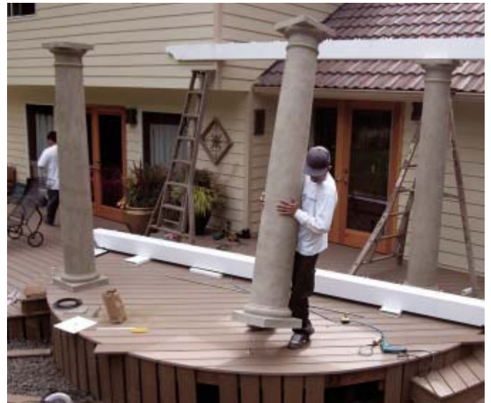
Figure 8. Fiberglass arbor and pergola kits are available to create a classical or Tuscan look. These hollow columns anchor to the deck framing using a length of all-thread.
